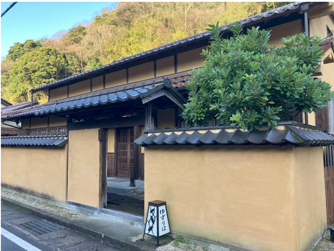
An old house restored as the “Yuzuriha” lodging facility
